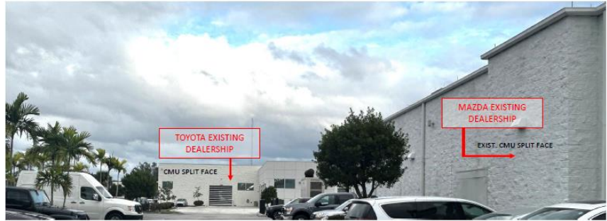
REAR ELEVATION / EXISTING IMAGES
